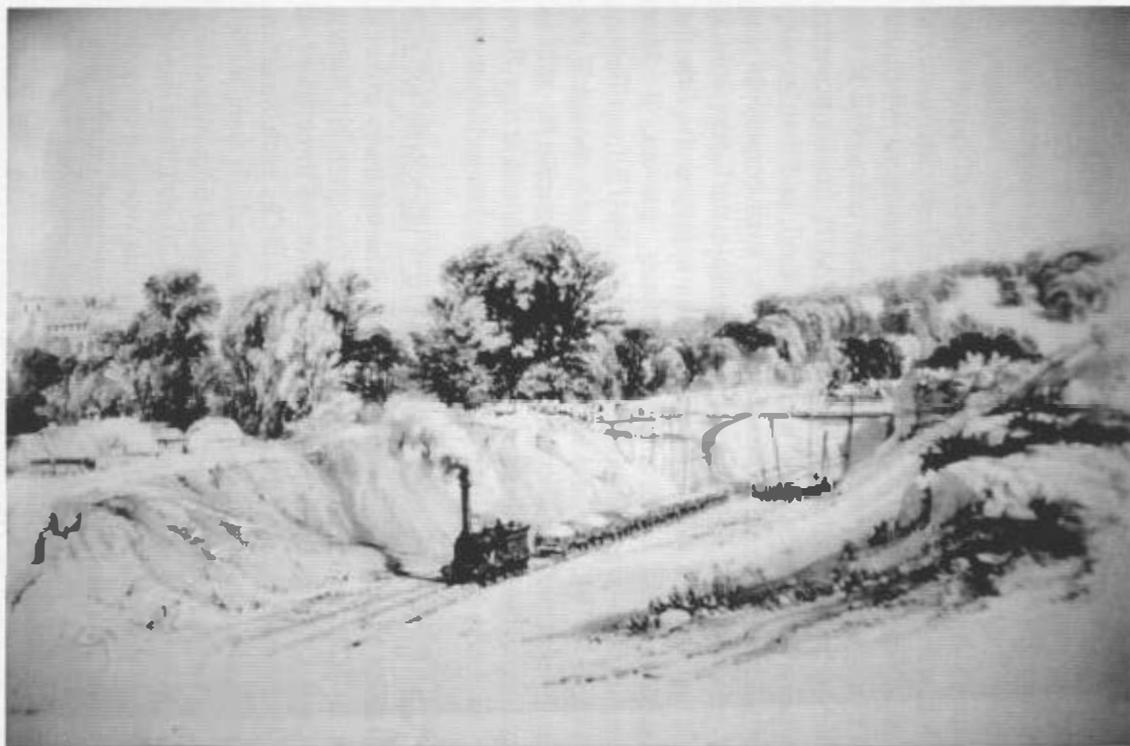
[392] The nature of railway construction before the introduction of steam excavators and high explosives in the 1880s. This view of the construction of Tiring cutting on what is now the West Coast Main Line comes from J C Bourne, *Drawings on the London & Birmingham Railway* (1839).
