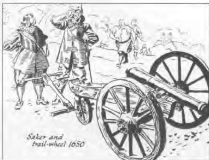
Saker, calibre of 3.5 inches, weighing 1,600 lbs, 3¼" calibre, wt of shot 6 lb.
